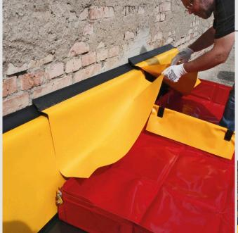
The metal body of the modular element is equipped with special rubber foam profile that seals the fixed joint of the drainage slot and the wall. Fluid removal is ensured by the highly resistant cover made of plastic coated fabric.
