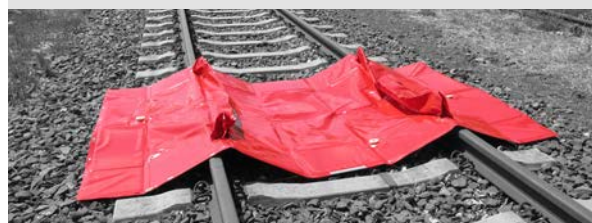
Folded out bund ready for final assembly
